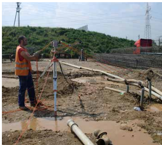
Performing of sonic trials on site
