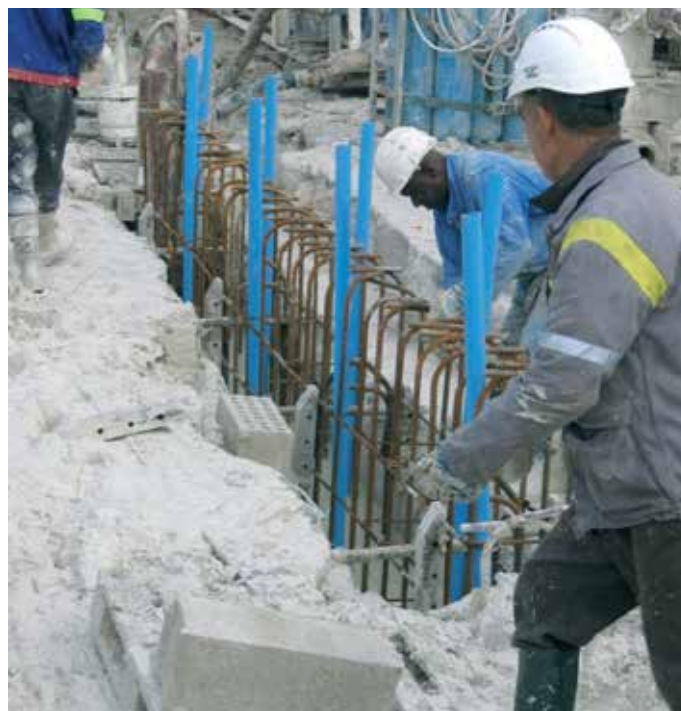
Reinforcement cage equipped with sonic log casings
